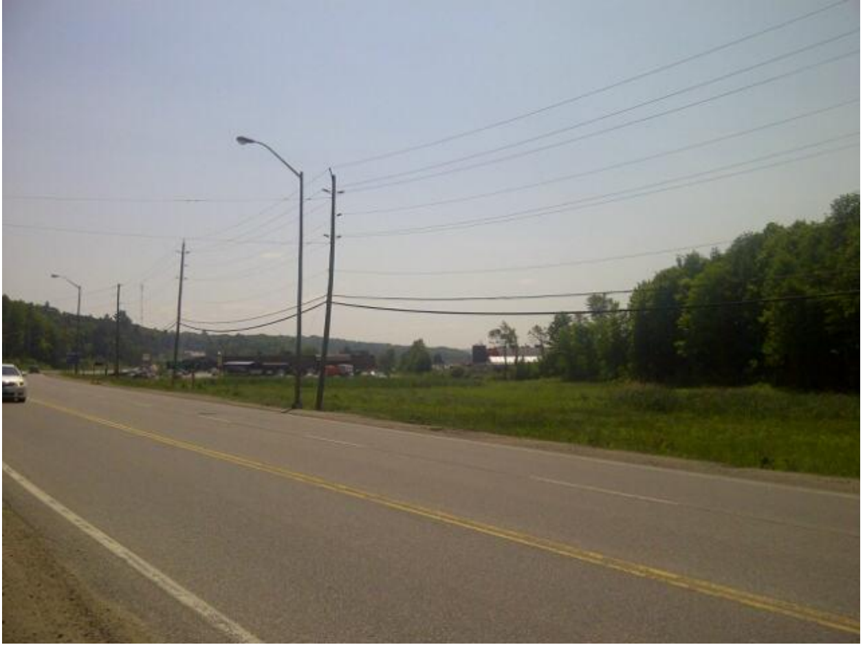
Figure 3 South-West view of the Future shopping centre site
